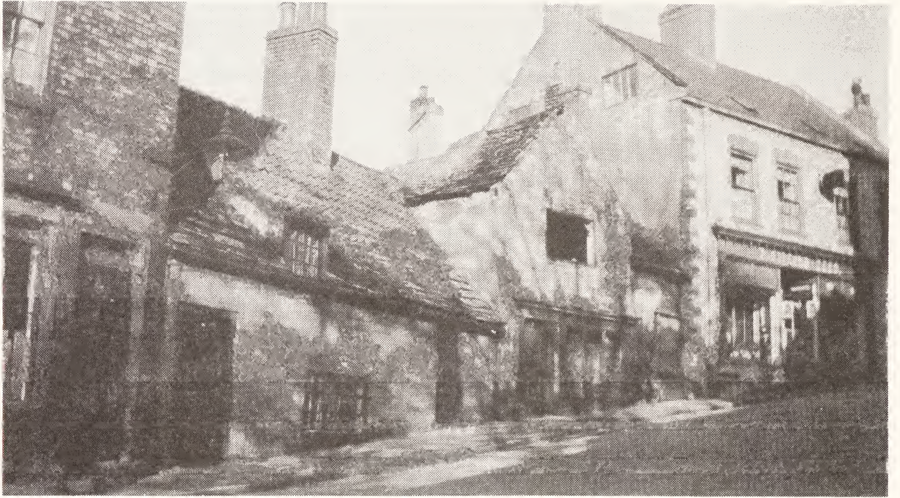
Plate 1. Nos. 5-10 Bedern Bank, Ripon, February 1935.
